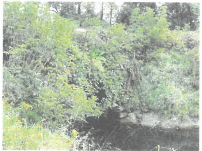
Upstream Culvert Inlet
